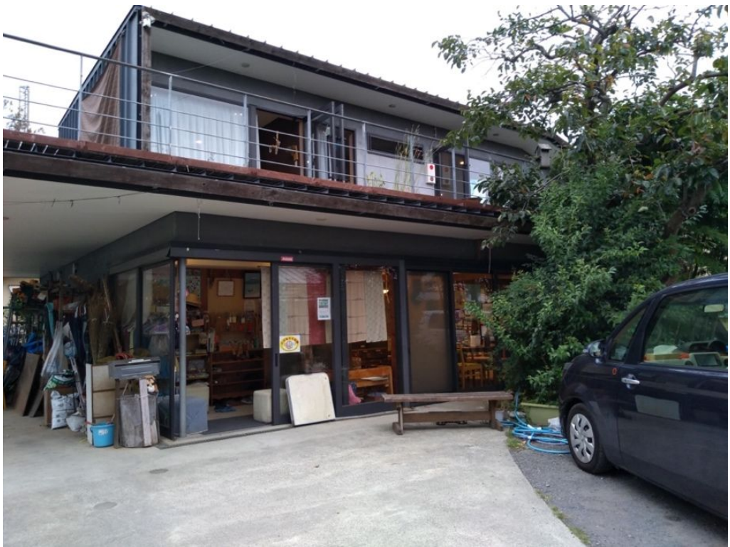
Photo 4. Aoi Care shared residential unit.
